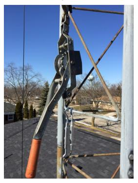
damaged leg. It surprised me of how much muscle I needed to put into the come-along to straighten it, but it worked. I placed the turnbuckles on the rungs and tighten them. For now I am viewing this as a temporary fix and need to devise a permanent solution which I can implement when the weather improves. I guess guying is a possibility.
