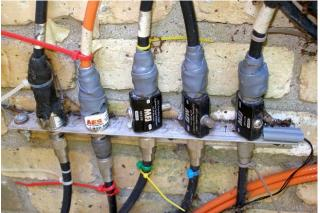
All the connectors are now protected with a drip loop in the co-ax and a caulk tape wrap to prevent any water ingress.
