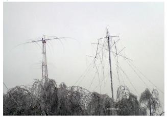
RD3A beam antenna following a freezing rain in Europe. Note that the ice overloaded and broke the trees as well as the beam elements.
