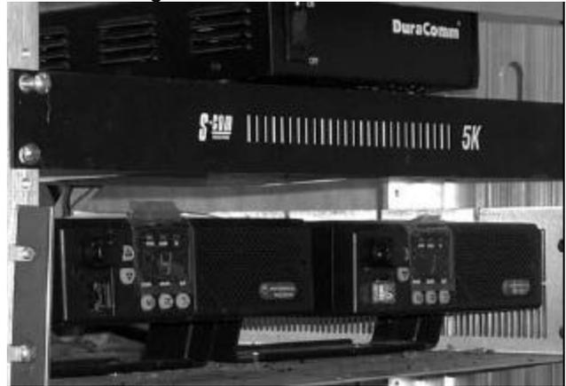
**The 5K Controller, Receiver and Transmitter at Remote Sites**
