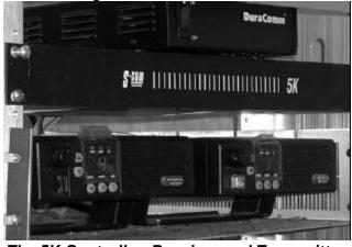
The 5K Controller, Receiver and Transmitter at Remote Sites
