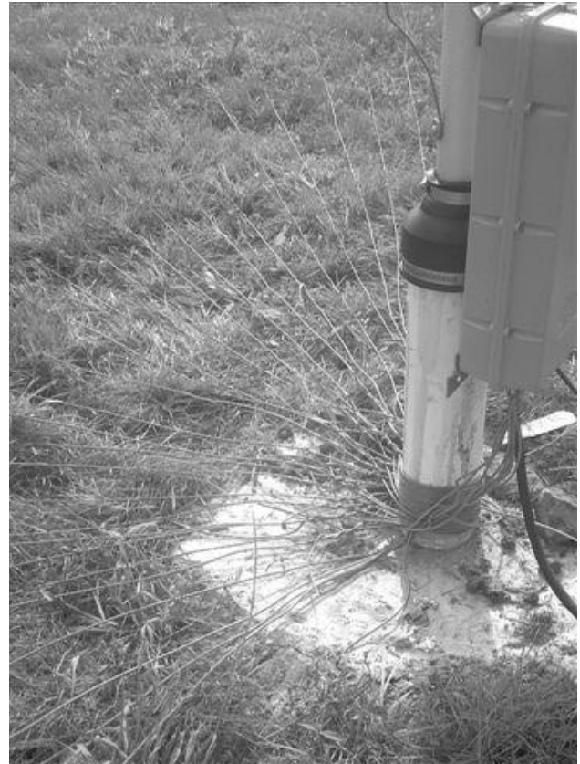
PVC Pipe Mount for Flag Pole Vertical Showing Termination of 120 radials at common ground rod
