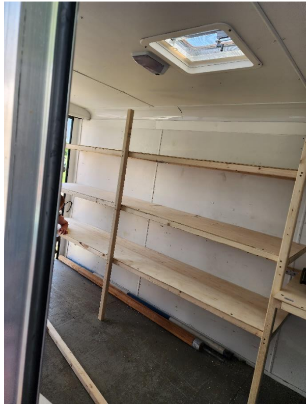
Trailer – Shelving Boards Added
