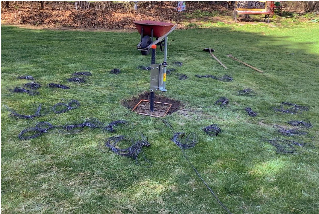
Center Pole Set – Radials Connected to Copper Tubing Base
