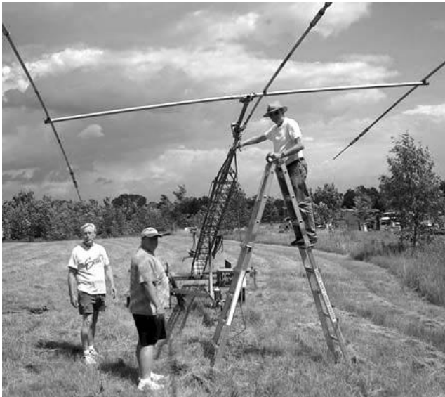
Steady as you go as the 15-meter team erects the trailer mounted tower & tribander under the direction of Leon, K9GCF
