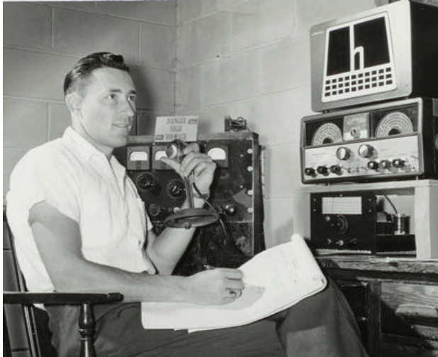
Here Ray is shown in about 1957 with his SX96 Hallicrafters receiver and his “home brew” AM transmitter using an 813 tube in the final. Oh for the glow of those filaments – transistors just aren’t the same.
