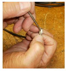
OK, it was now time to solder the coax to the tubing prior to cable-tying it to the mast. Because of the required length of the shield and the center-conductor separated by the mast, I decided to pull the center-conductor out of the braiding. If you haven't seen it done, all that is needed is a sharp tool. Start by putting a sharp bend in the coax at the point where the jacket is re-
