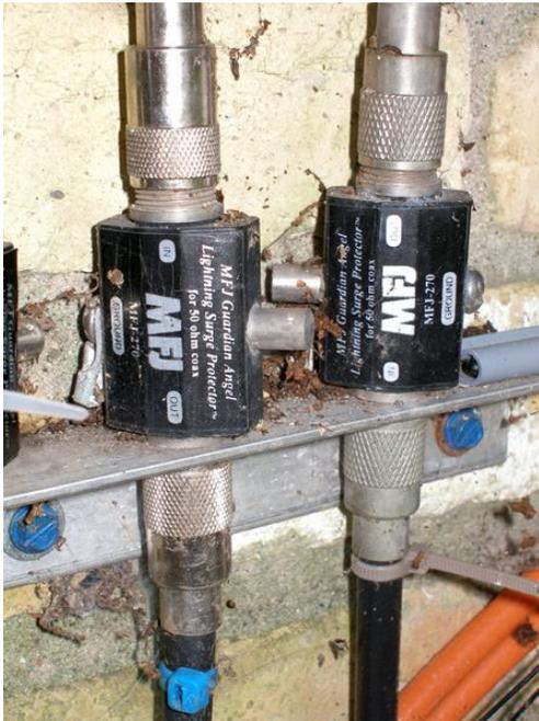
**The lightning arresters are fed through a grounded aluminum angle iron for secure protection.**
