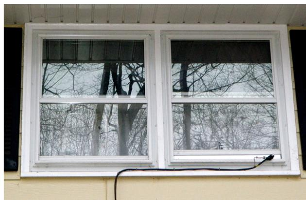
Then a wood spacer was cut to install in the lower portion of the inside window frame. Three 3/4" wide slots were cut in the wood spacer and then 1/2" adhesive backed weather strip was inserted into the slots to form a slit and seal the area through which the antenna coax and ground wire would pass.
