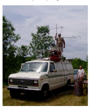
Ken Boston (W9GA) was busy attaching the 2 meter and 70 cm antenna to the OZARES communications van mast under the supervision of Todd Sprinkmann (KC9BQA)
